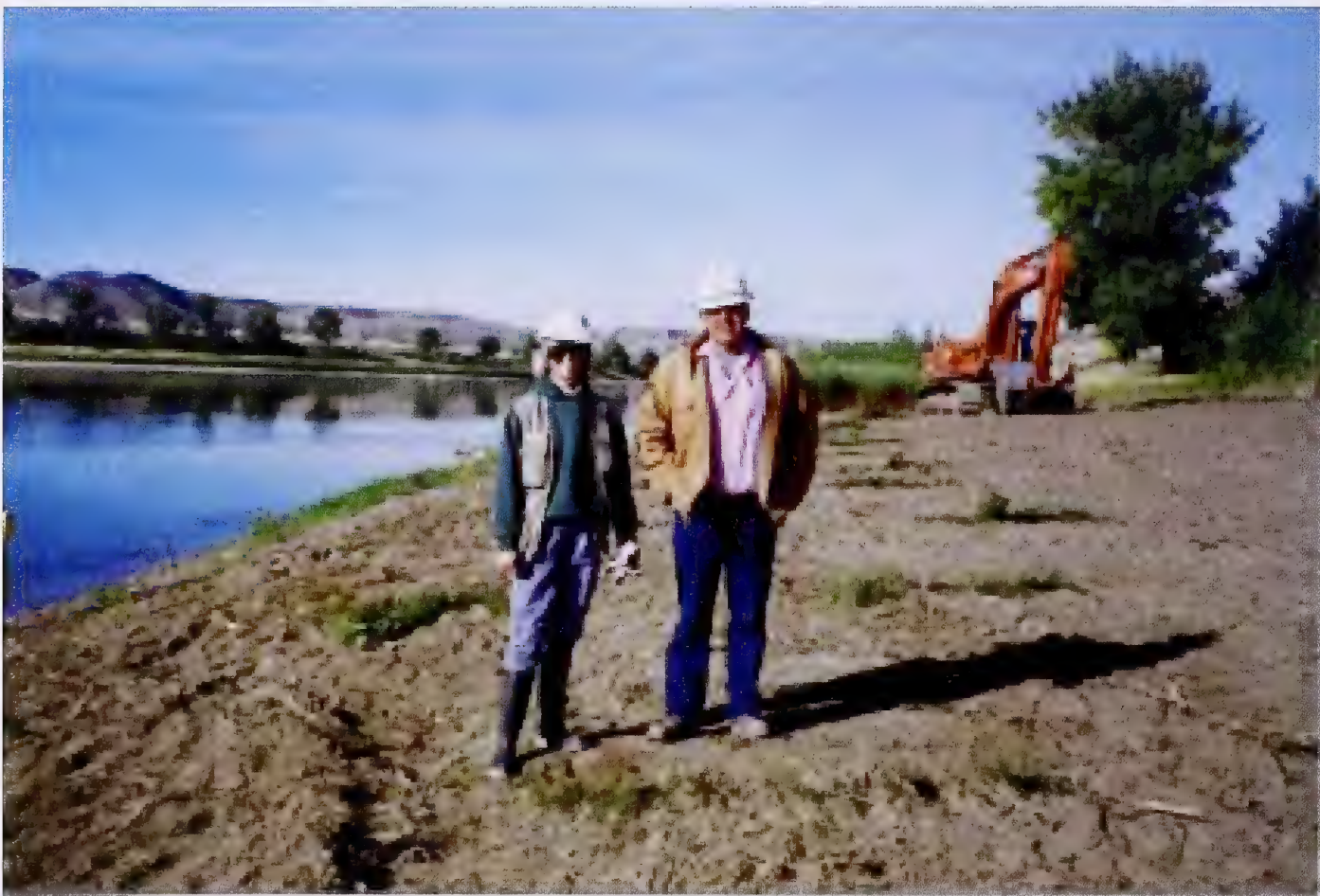
Photo 2 Express Pipeline - South Saskatchewan River Crossing.
